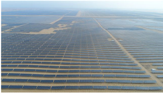
(a) Photovoltaic power station in the Kubuqi Desert.
