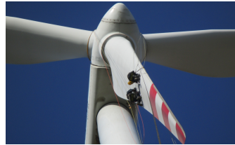
(b) Maintenance personnel are repairing a wind turbine blade.
